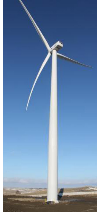
The college’s 1.65-megawatt wind turbine is located three miles north of LRSC.
